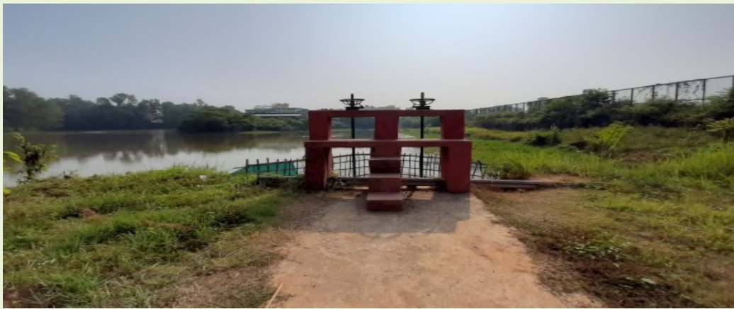
Fig 4: Sluice gate for sustaining and controlling flow/water level of the University Lake
